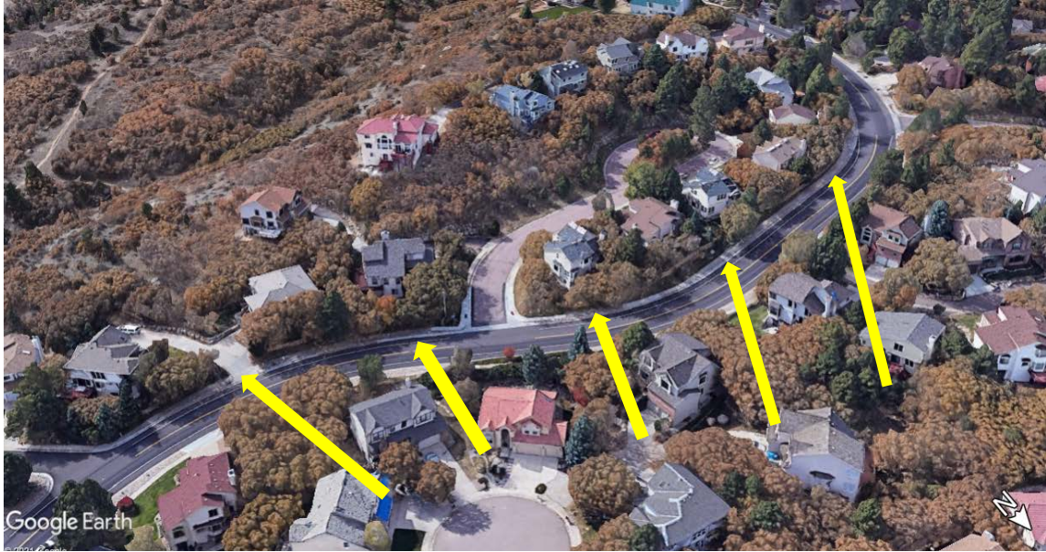
Figure 9 - South Side of MOHA Owned Fencing / Curbing Along BBD (Fencing Phases 2 & 3)
