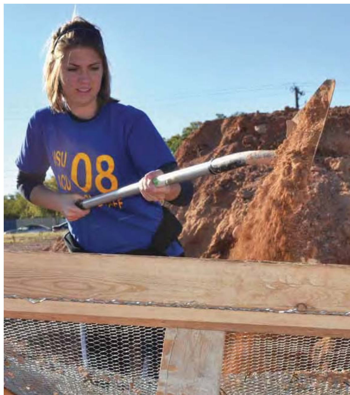
LEFT Lydia Vanderstoep, a Hardin-Simmons University senior majoring in Spanish and education, works on making slurry at the Friendship House construction project. The slurry is used for the earthen brick homes on the city block that makes up the Friendship House complex. Lydia has logged more than 200 hours of community service since she came to HSU three years ago. BELOW LEFT HSU student Shannon Rector, a junior elementary education major from Abilene, applies mud to the walls inside one of the earthen houses. Houses will be sold to low-income residents who qualify and will surround a park/playground when the complex is complete. OPPOSITE PAGE Volunteers and contributors have helped make the North Park Friendship House a success.
