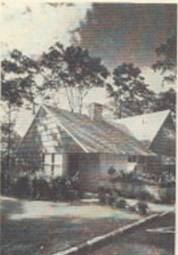
All-weather driveway is paved and curbed
