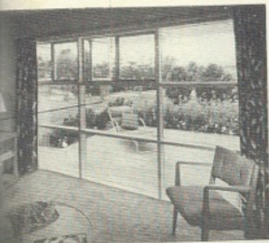
Living-room bay, 7' x 12', views garden and terrace. Wood frames support insulating-glass panels, each 25" x 45", and aluminum sash.
