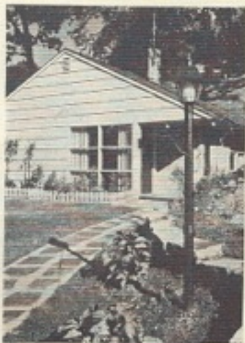
6-foot overhang shelters the front door
