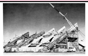
The second addition to Irvin High School of 1961-62 was 40% complete as shown in this picture. The new construction, located west of the main building, housed facilities for physical education, band, and ROTC classes beneath the stadium seating.
