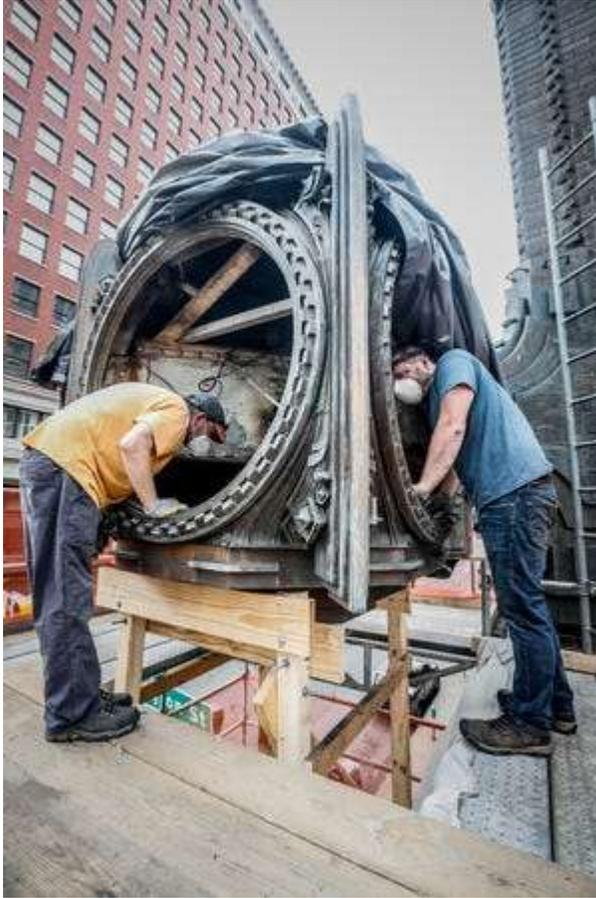
But during the 2016 restoration, Klinkose noticed the rust on the clock and that it was leaking water.
