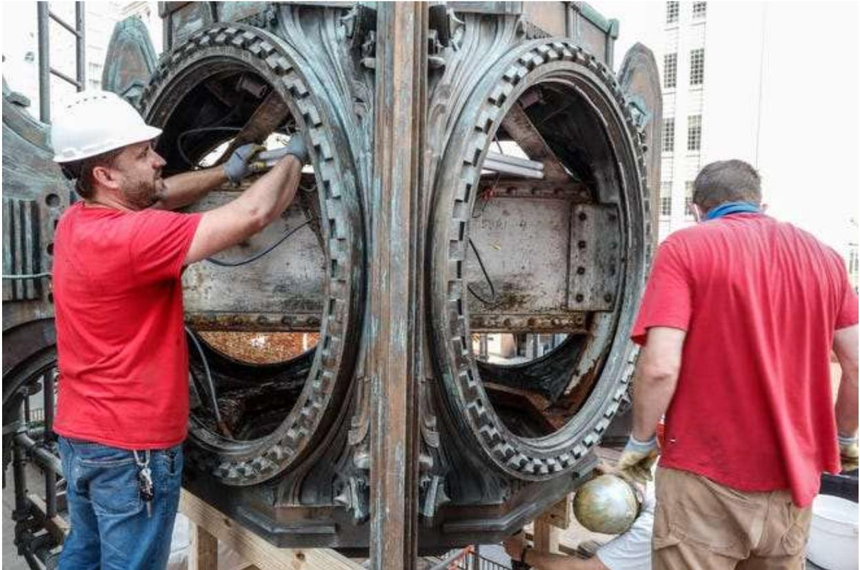
While the bronze encasing the clock has turned a bit green over time, Klinkose said it just needs a good scrub. The tough part will be the water damage and rust on the steel armature or frame inside the clock.
