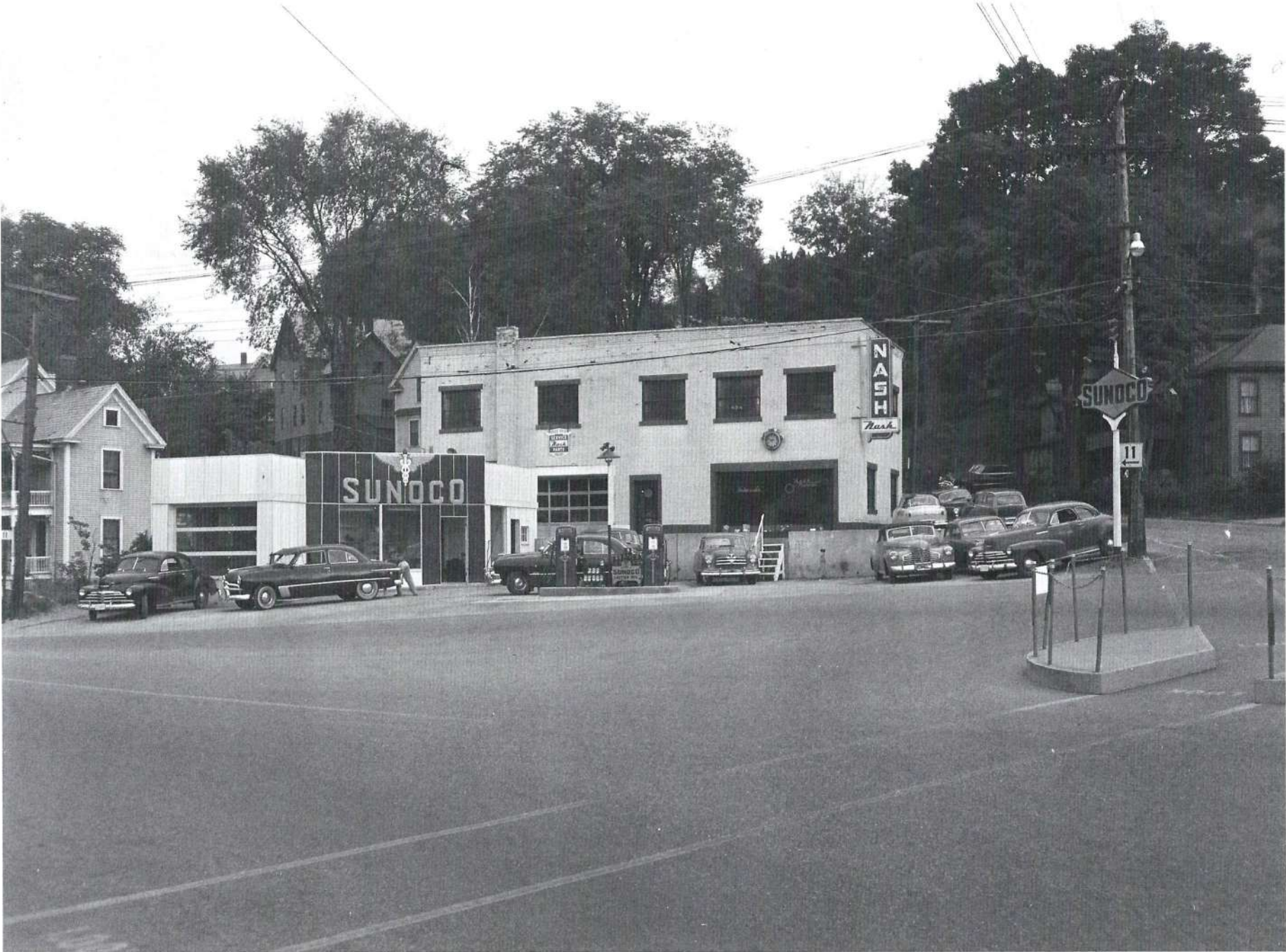
Sunoco-Nash Garage Clinton St.
