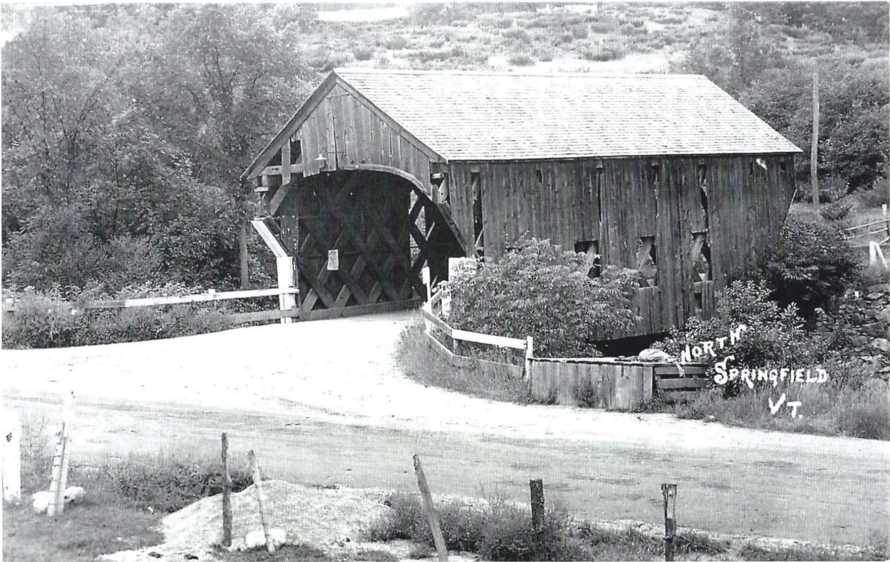
Baltimore Bridge North Springfield
