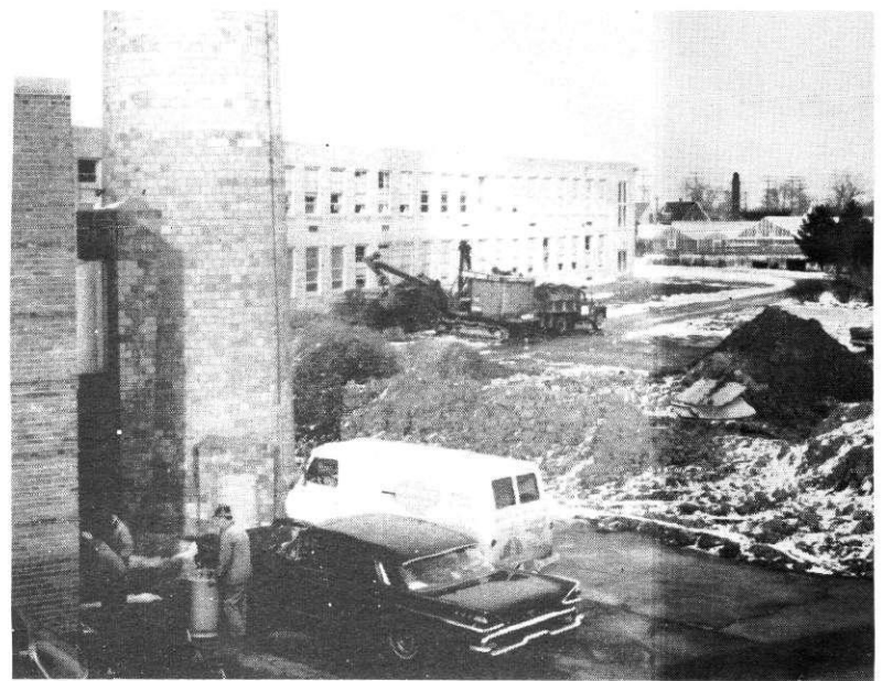
ABOVE: Shovel digging foundations for east wall of new wing. Present boiler house at left. BELOW: New Board of Education maintenance garage to left of present shop wing.
