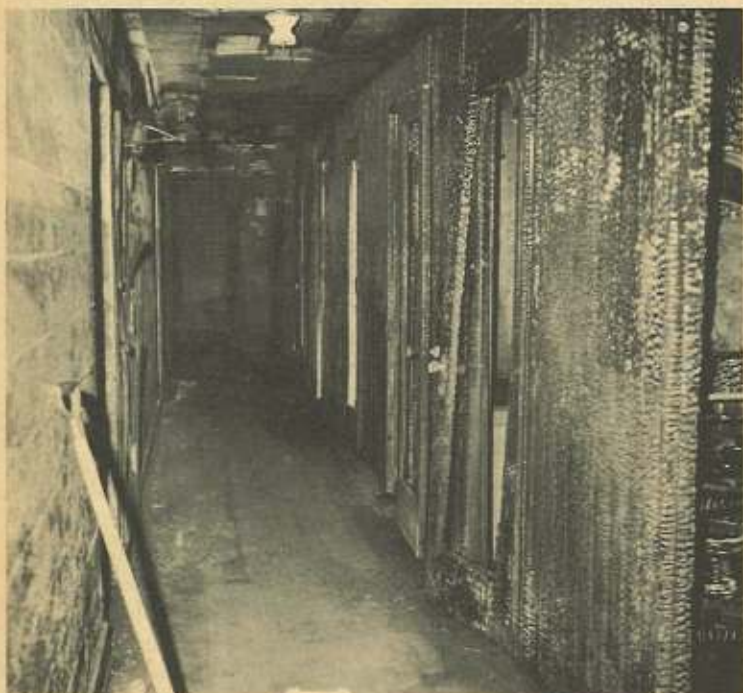
An aftermath of the halls and dressing rooms charred by fire. (OLE PHOTO)
